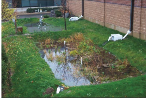
Figure 7. Side-by-Side Rain Garden Configuration
