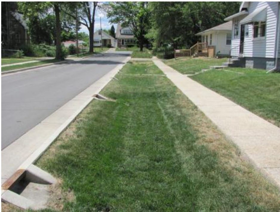
Figure 6-1. Bioretention Planted with Turf Grass
