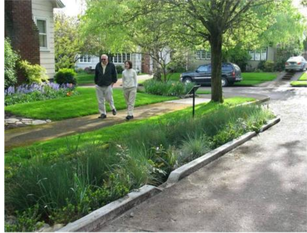
Figure 4-2. Curb-extension Bioretention
