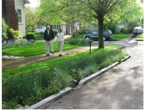
Figure 4-2. Curb-extension Bioretention
