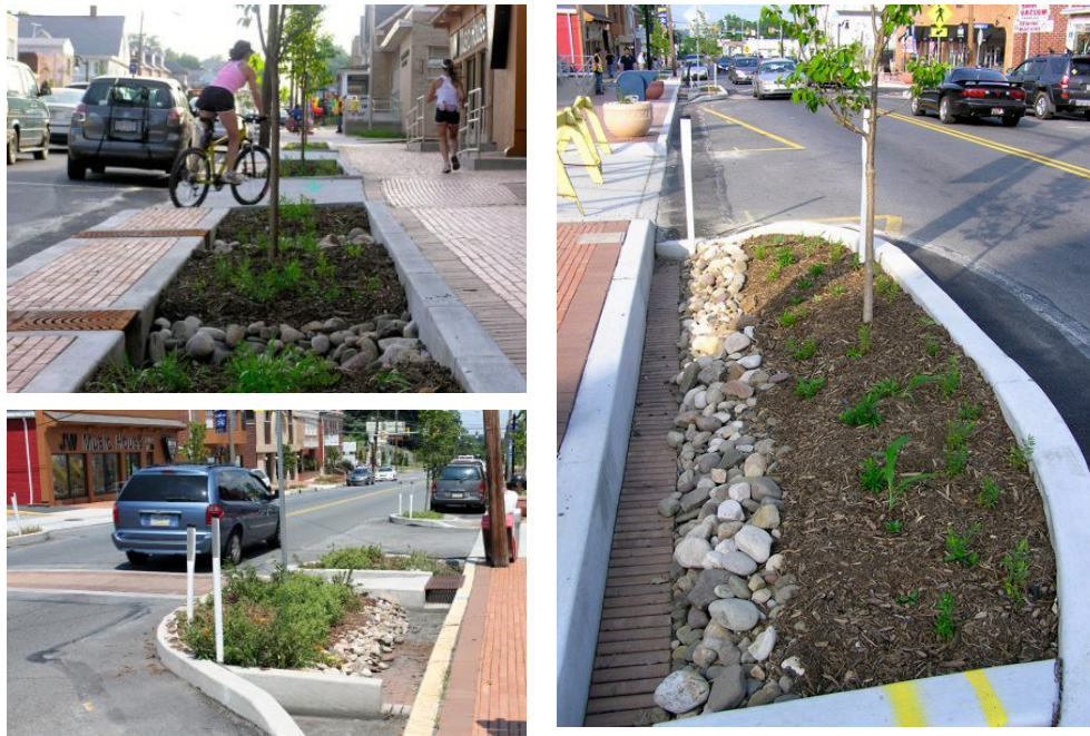
Figure 16. Lemoyne, PA Market Street Rain Gardens
