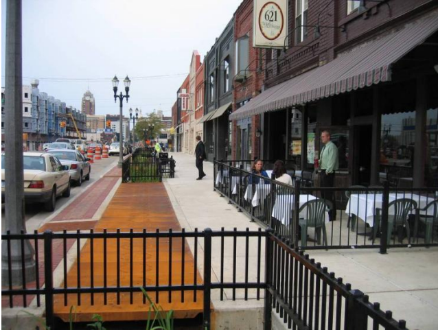
Moveable metal plates over bioretention providing for outdoor seating.
