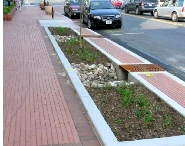
Metal plates allowing pedestrian access from roadside parking.
