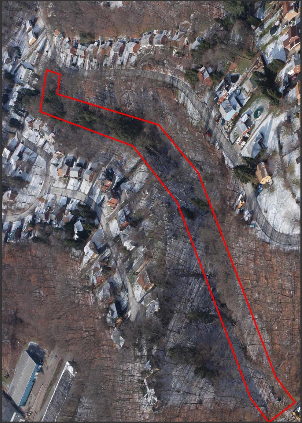
Willet Road Project Area – Pre Construction Photo
