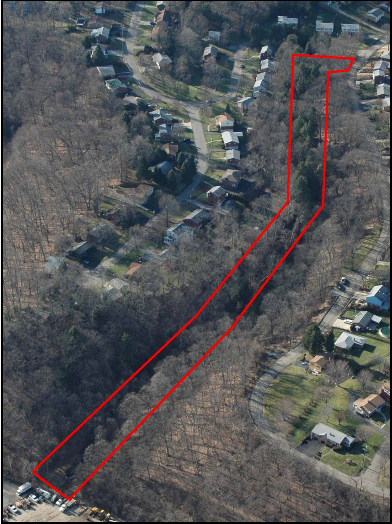
Willet Road Project Area – Post Construction Photo
