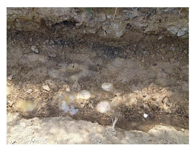
Poor site management causes big problems. This rain garden on a construction site being used as a lay down area during the winter.
