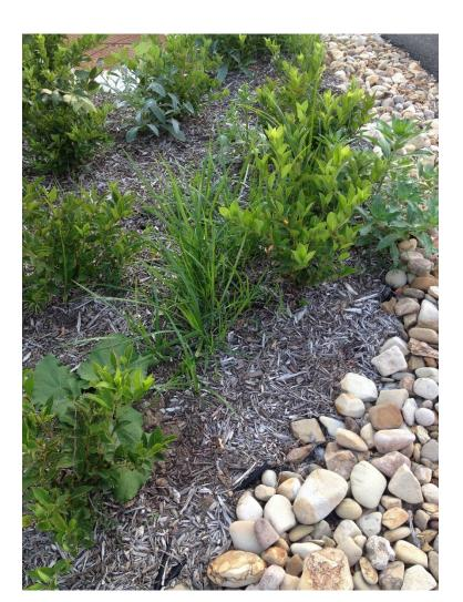
Rain garden short circuit and excessive siltation from parking lot run off. Not enough water is going to get into this rain garden to do any good.
