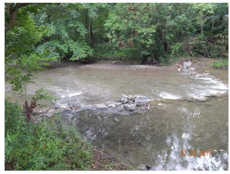
Constructed from riprap, created 2 streams, rock unstable and pushed downstream after a storm
